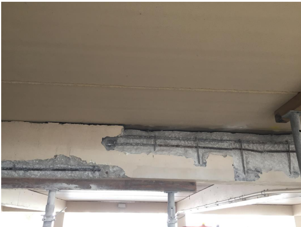
Picture 2: In-progress concrete repairs
