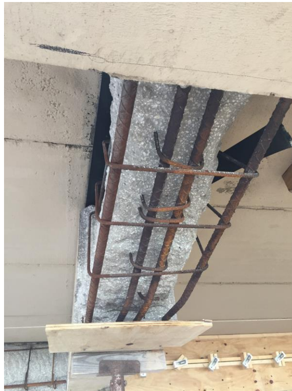
Picture 4: Approved concrete excavation
