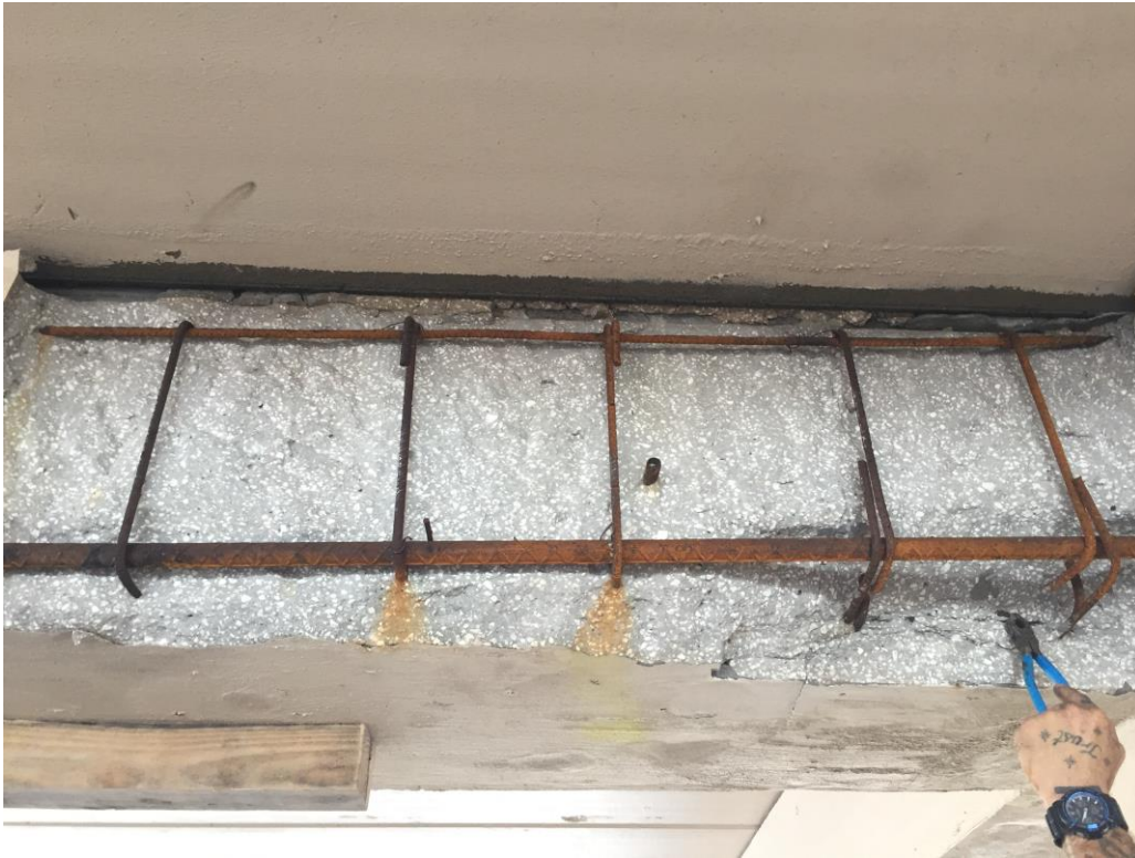
Picture 1: In-progress concrete repair
