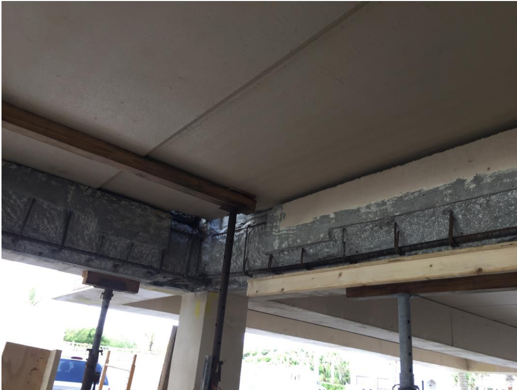
Picture 3: Approved concrete excavations
